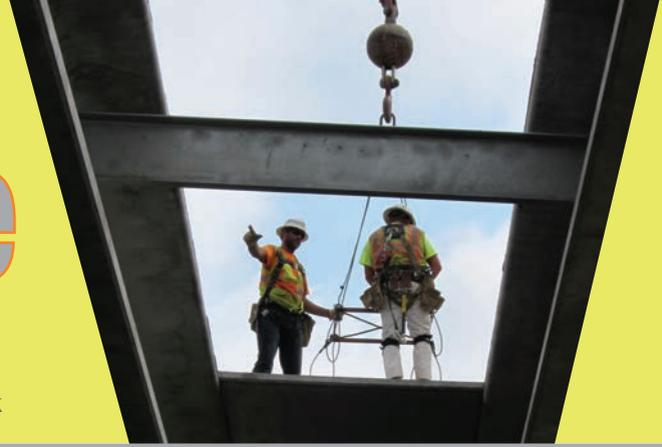
Just east of Jefferson City, Mo., sits a construction site that recently became home to one of the nation's first bridges to incorporate an unusual concrete mix in its girders and support structure. The three-span bridge, which was completed this fall on Highway 50, is outfitted with various sensors and instrumentation to collect data on how well the bridge performs over time.
